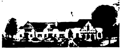
The Community House at Longview, Washington; modern in every detail, open November, 1923
